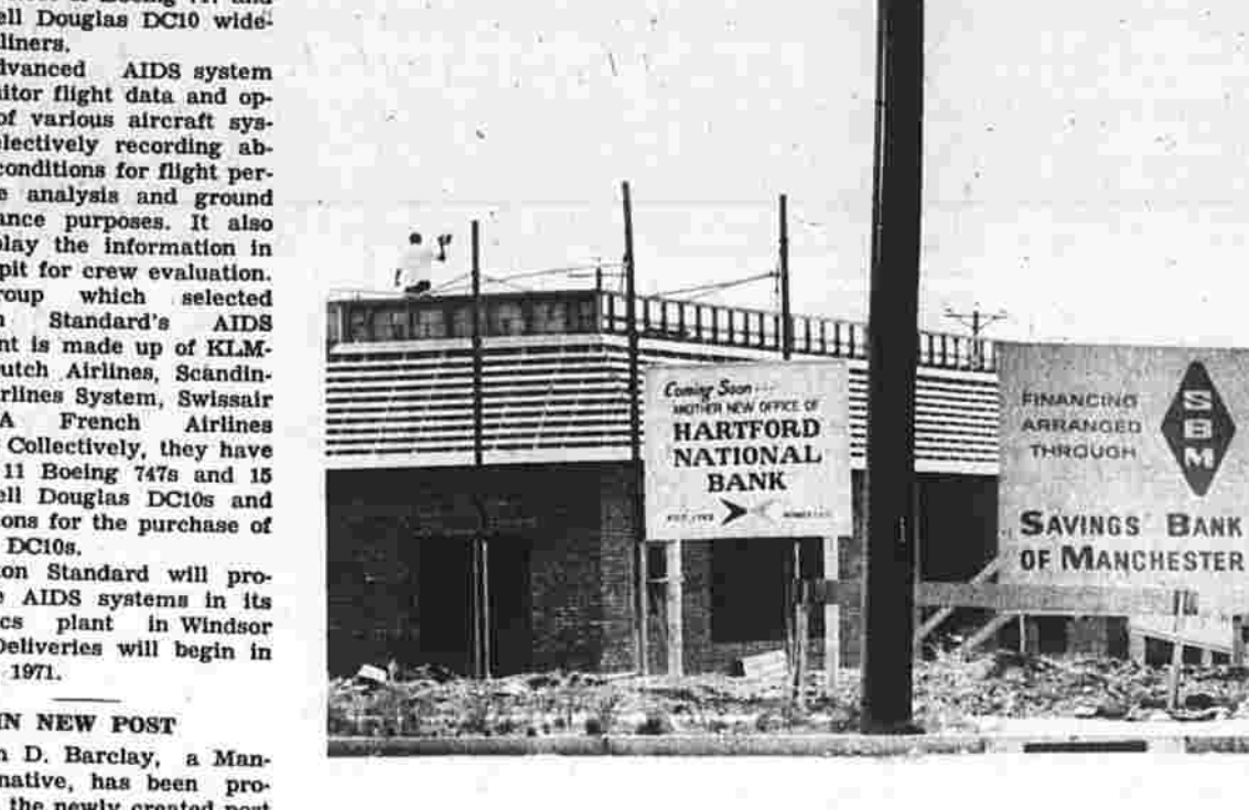
Everybody knows money's scarce and costly to borrow these days. But despite the implication of these signs, Hartford National is not really financing its new offices through SDB. The building is the store block at Main and N. Main Sts. in the North End Redevelopment Area, where both banks will establish branches. The block's key occupant will be a Top Notch Foods Supermarket.
